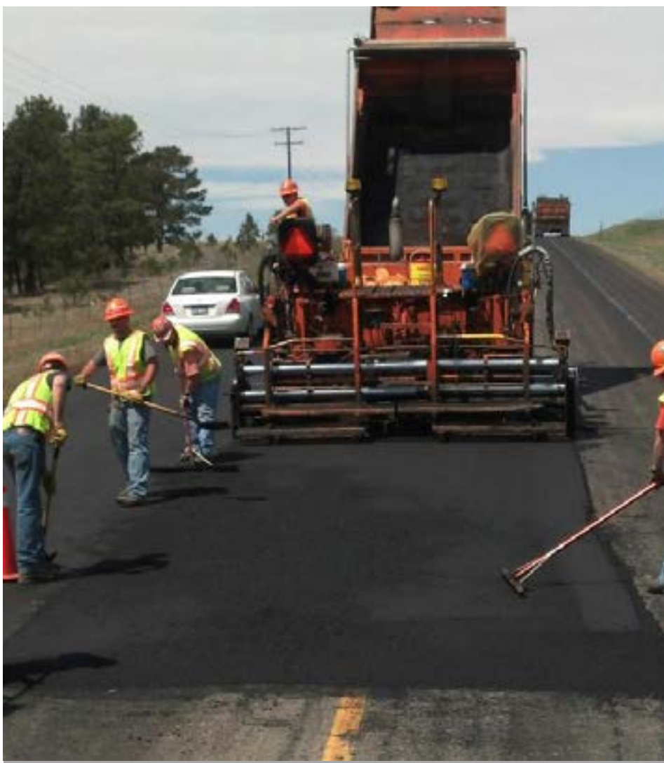
Construction on US 287 in Lamar.
